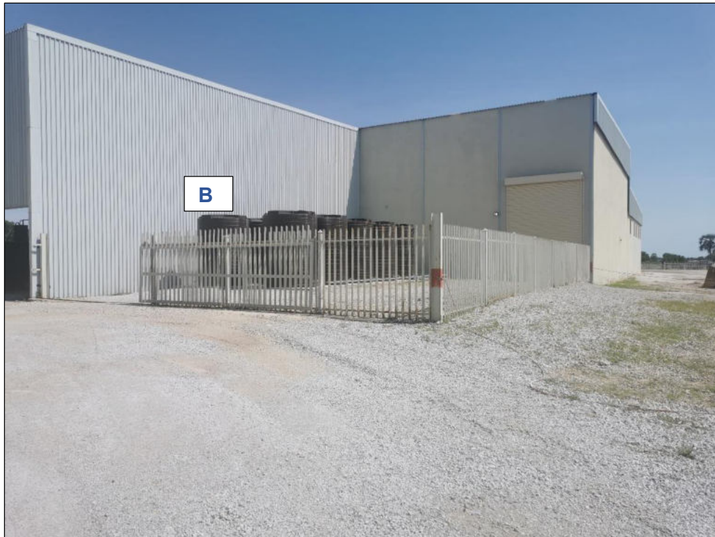
Figure 2-5: A- the 8 water tanks for the office and B- factory use water storage tanks onsite
