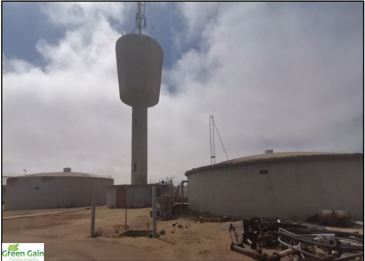
Figure 9: Overview of the existing bulk water storage facilities
