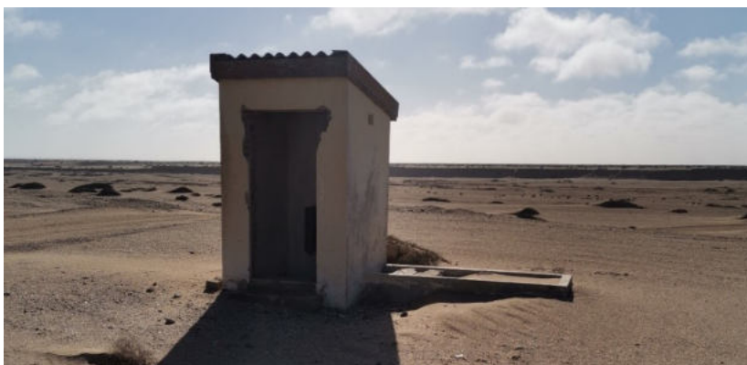
Figure 6: One of the three boreholes not in use
