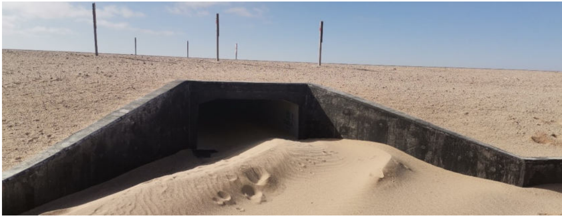
Figure 2: Existing culvert on the C34 road
