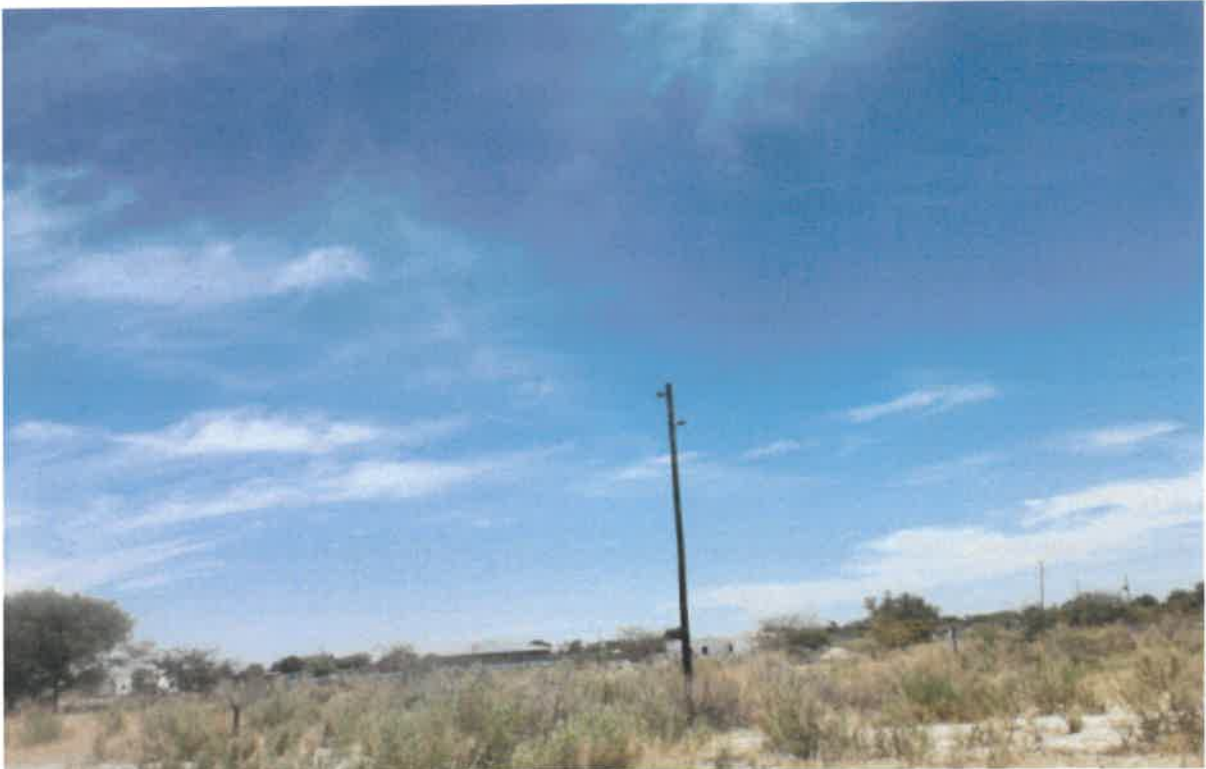
Figure 6: Existing electricity infrastructures (powerlines) in the area (HEEC, 2022)
