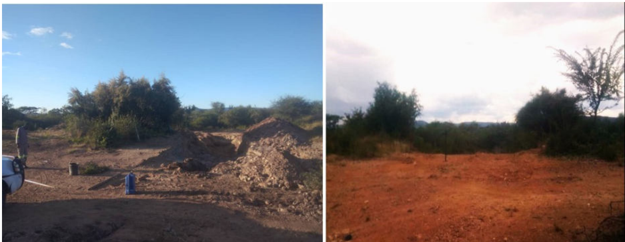
Figure 6. A Trench before and after backfilled
