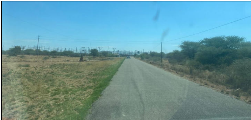
Image 1-5: Paved access from B1 turnoff
