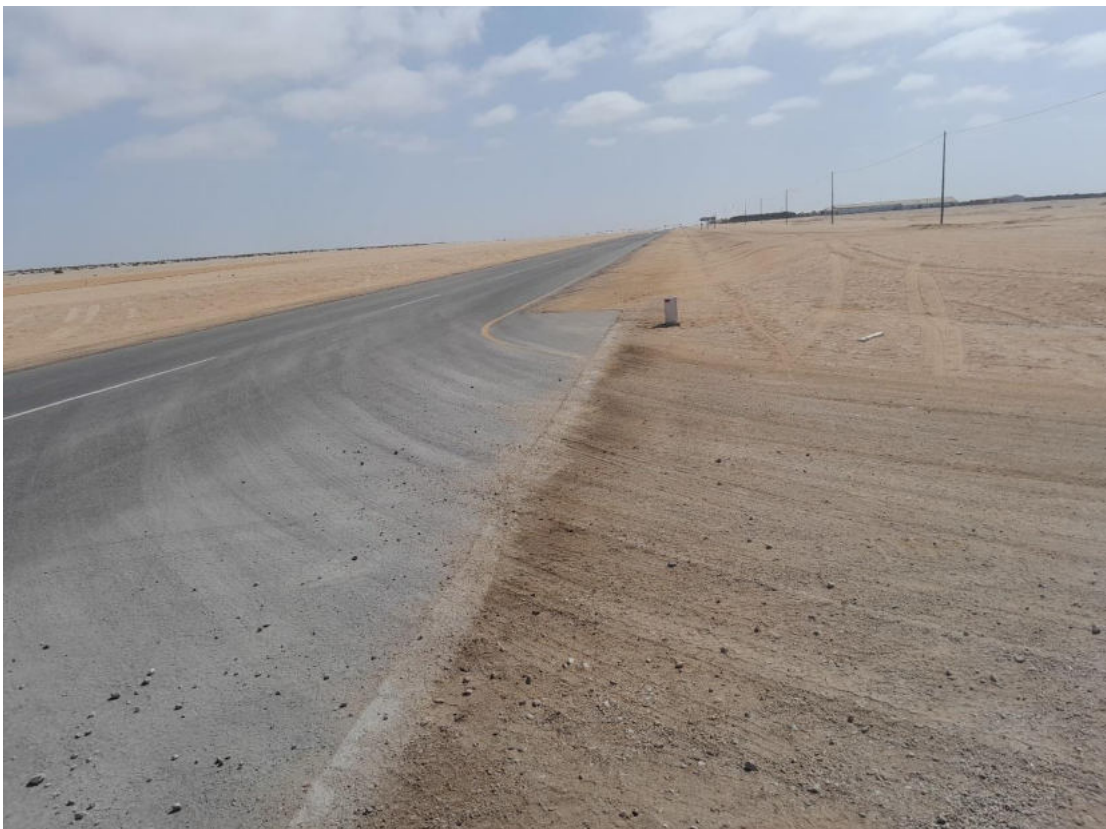
Figure 12: Access to project site: Henties bay-Usakos tarred road
