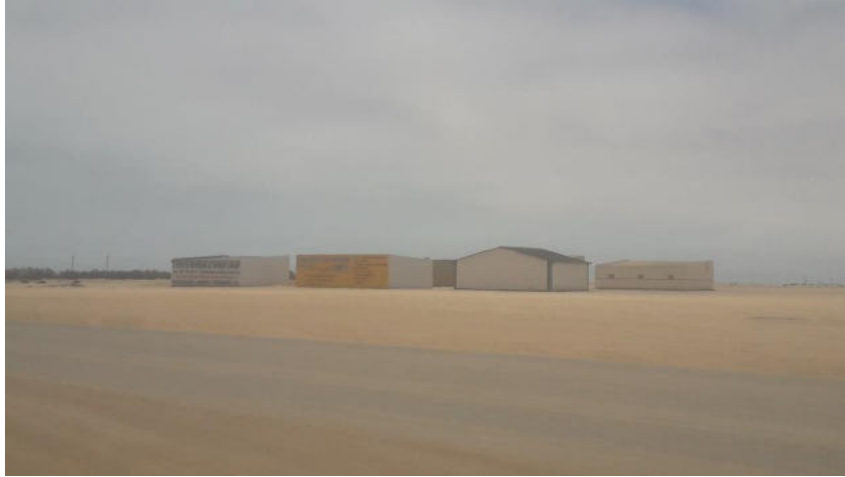
Figure 18: Existing aircraft hangers within the Henties Bay Town Land no. 133
