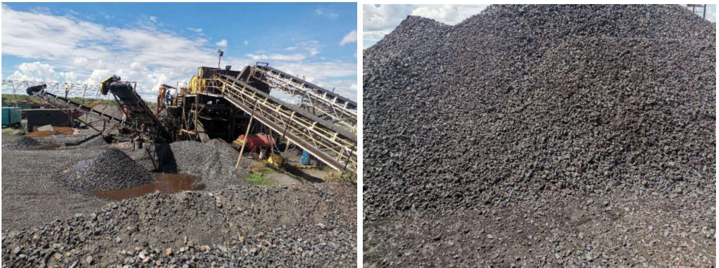
Figure 6: Manganese processing plant at Otjozundu mine
