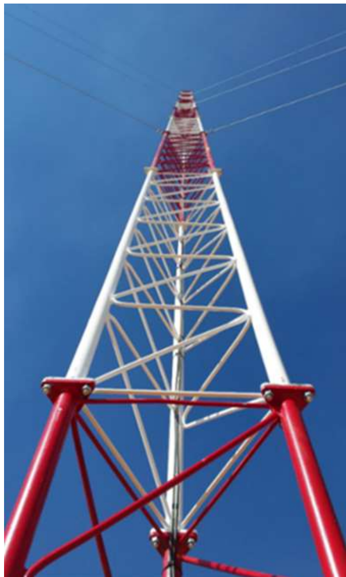
FIGURE 6-2: STEEL GUYED LATTICE MAST SECTION
