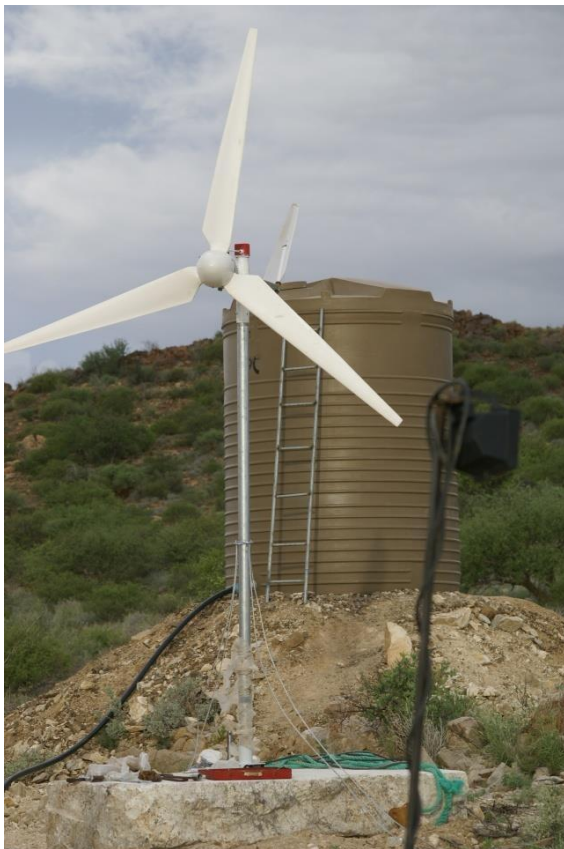
Figure 8: On site temporary infrastructure such as the wind power generator and water storage tank
