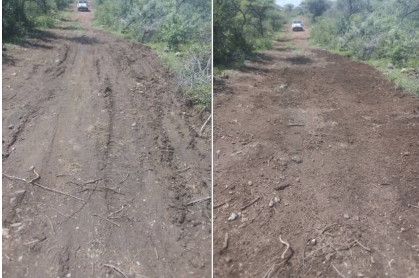
Figure 5. Track to access road before and after rehabilitation
