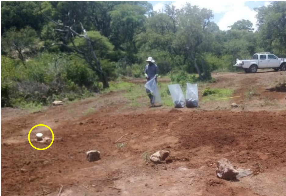
Figure 4. PVC casing cut to the ground and capped
