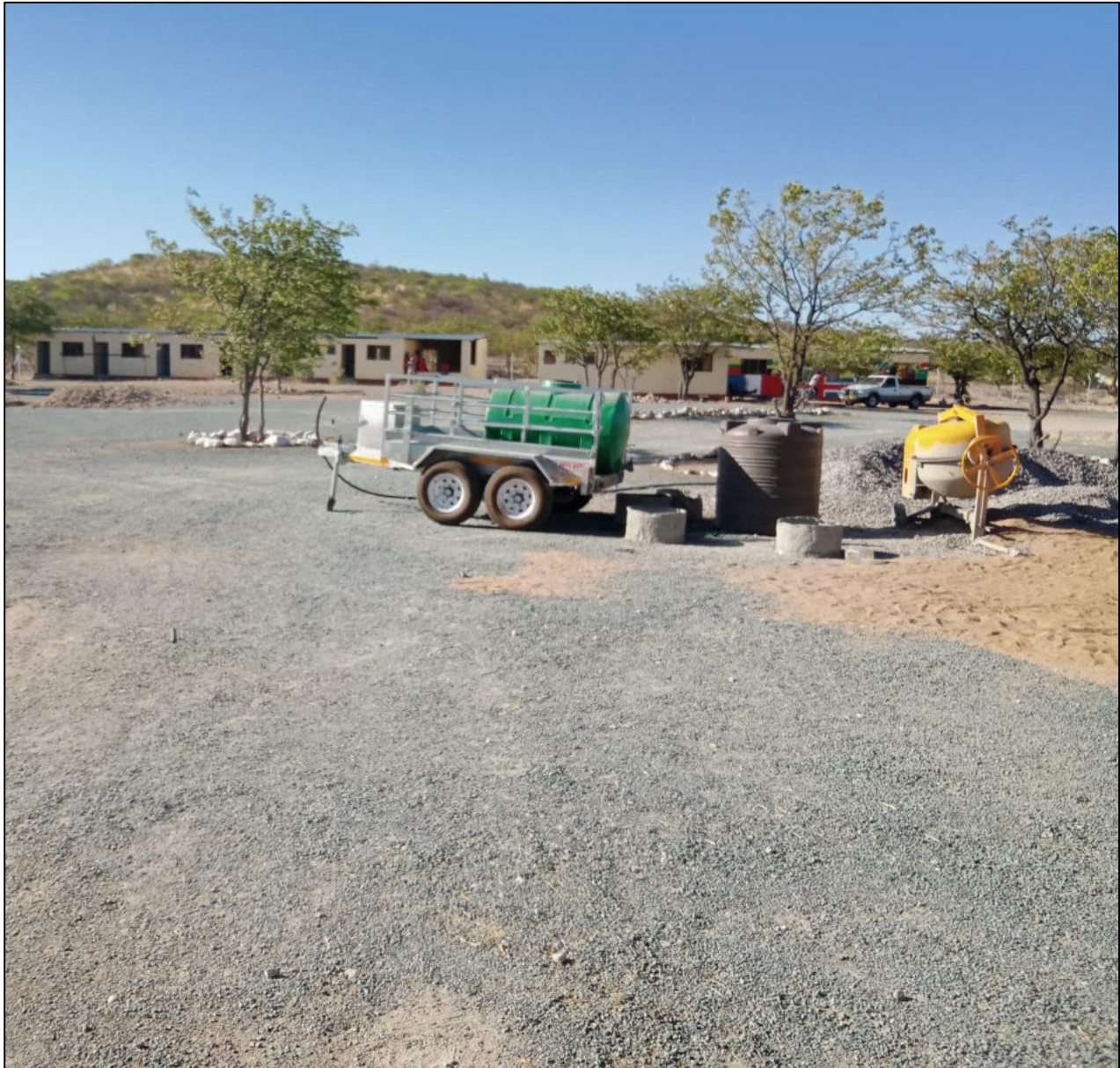
Figure 2: Shows a block of one of the existing staff accommodation on site.
