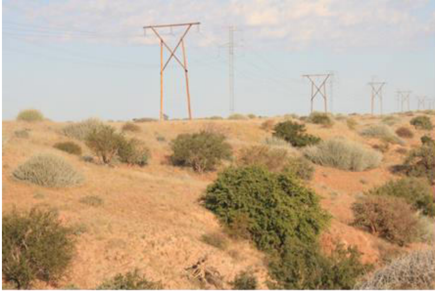
Figure 3. Well vegetated and rocky areas in the general Khan Substation area.
