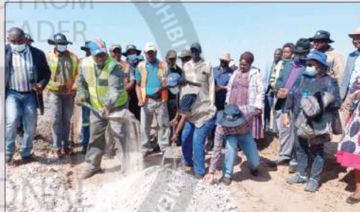
New beginnings... Works minister John Mutorwa and Kavango West governor Sirkka Ausiku break ground to begin the construction of the Charlie Cutline road at Casava village on Thursday. Photo: John Muyamba
