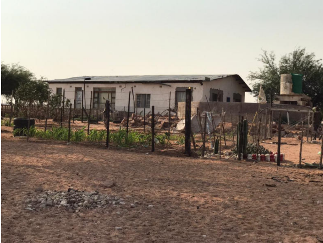
Figure 15 a dwelling / house observed on site
