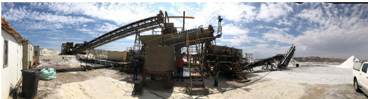
Figure 3. Image of the processing plant captured in April 2021. Source: (L. Amwele, 2021).
