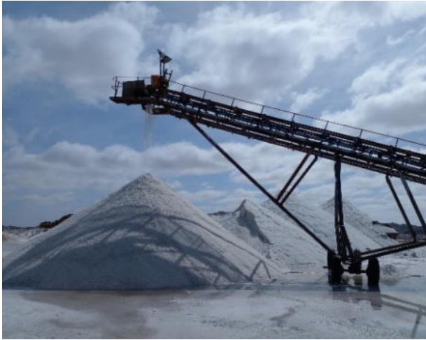
Course salt product drying stockpile
