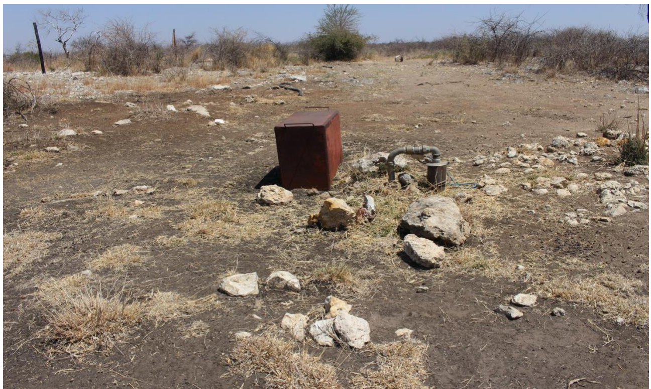
Figure 6: Water supply borehole on site.
