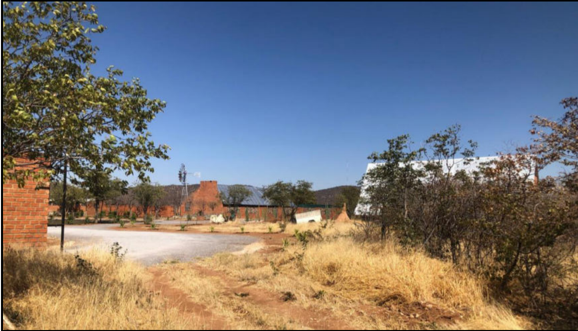
Figure 3: Infrastructure on site
