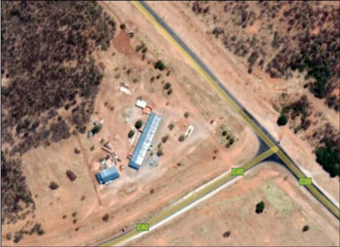
Figure 4: Photo showing the 4x4 fitment centre and restaurant/conference facility
