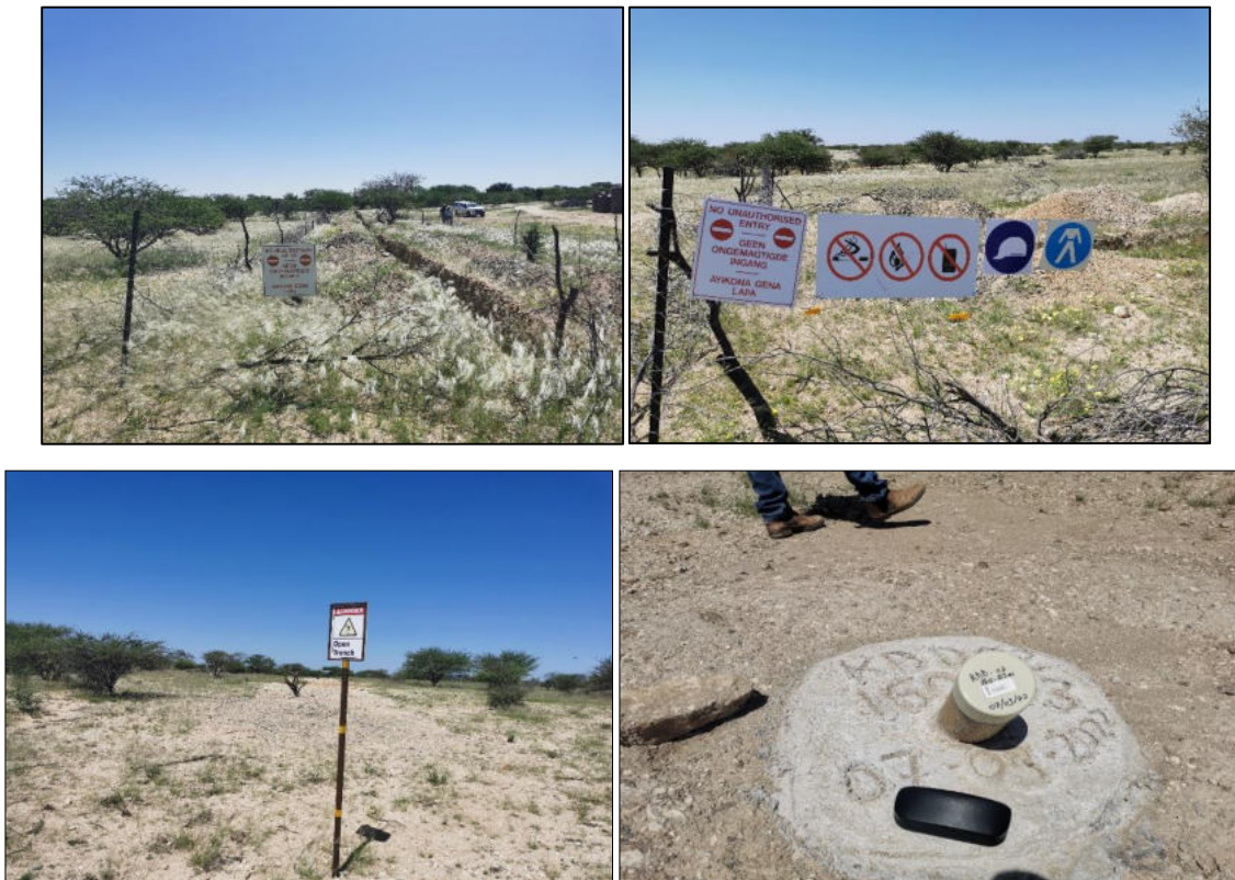
Figure 2-7: Fenced off exploration trenches awaiting backfilling upon completion of sampling (photos recently taken by Author at an active EPL visited by the Author near Okombahe, Erongo Region
