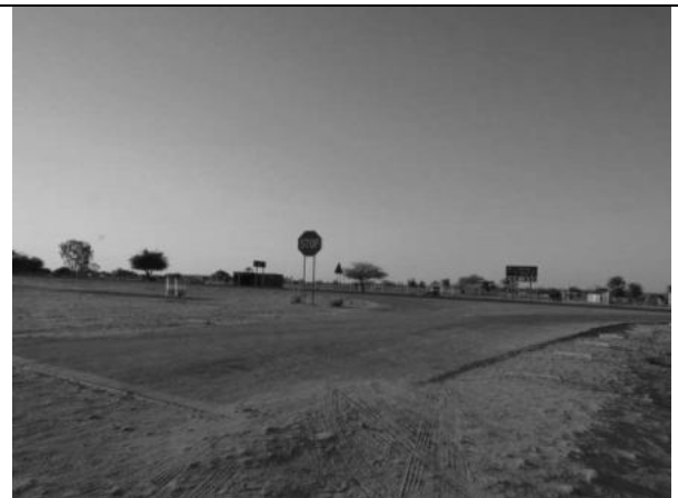
Figure 4: East- junction of C46 main road of Outapi-Ruacana and Etunda Irrigation Scheme
