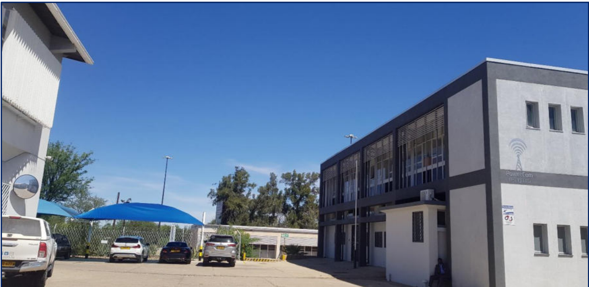
Figure 7: Building No. 3 (PowerCom Offices and Parking Bay)
