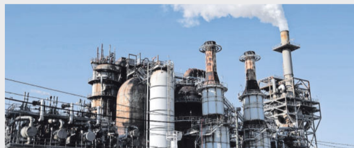
The LyondellBasell refinery, located near the Houston Ship Channel, is seen in Houston, Texas, U.S., May 5, 2019. PHOTO REUTERS/LOREN ELLIOTT
