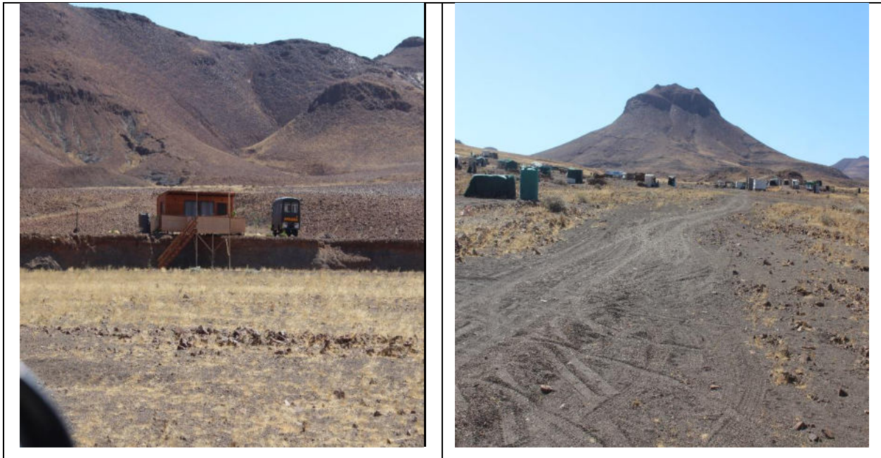
Figure 15: Show some infrastructure found within the EPL area
