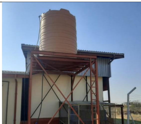
Photo 4-8 Existing water storage
