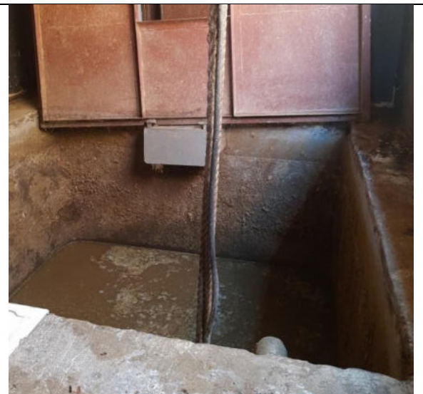
Photo 4-10 Effluent collection (to be demolished)
