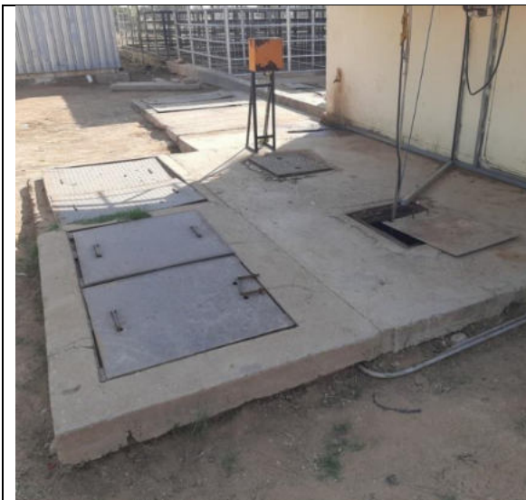
Photo 4-9 Existing collection (to be demolished)
