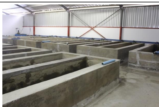
Photo 11. Wet storage tanks
