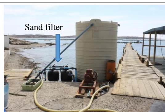
Photo 12. Seawater supply system with sand filter
