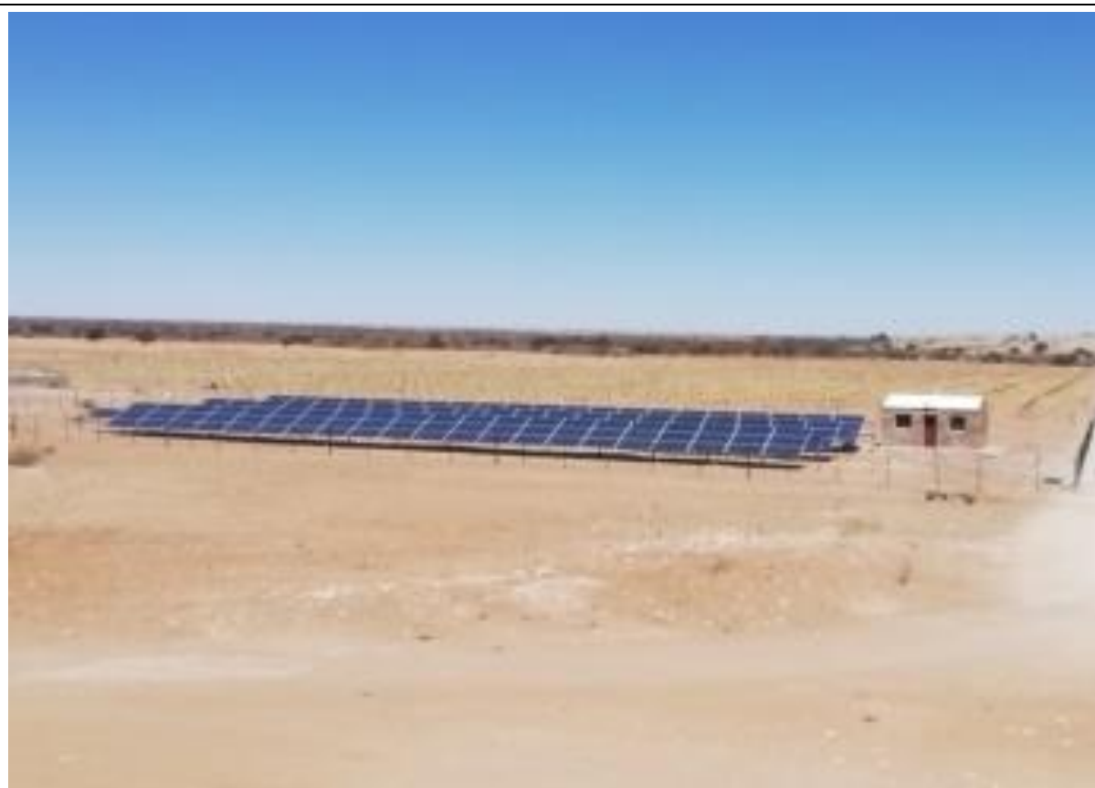
Photo 12. 48 kW Photovoltaic plant with pumphouse
