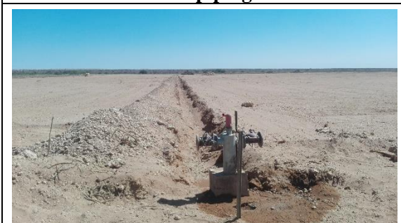
Photo 3. Installation of pipelines and related infrastructure
