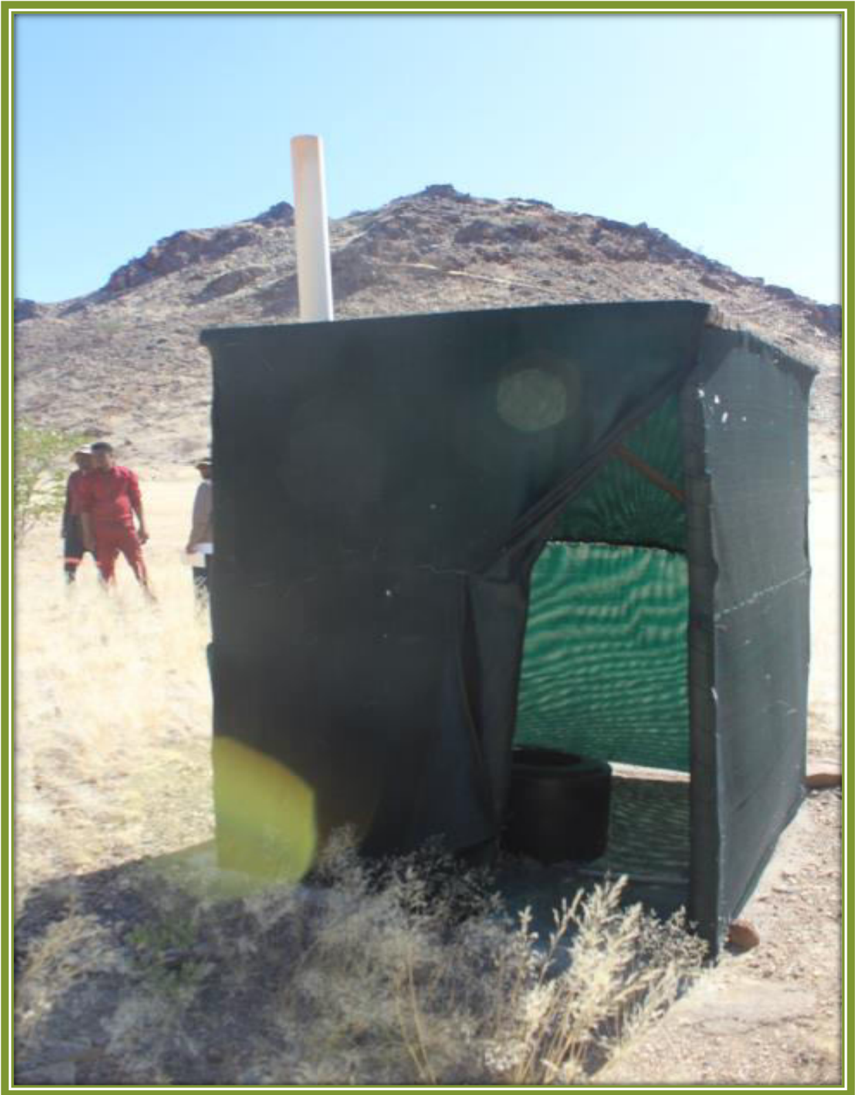
Figure 6: Existing toilet facility in the area of the mining claims used by the local artisanal miners.
