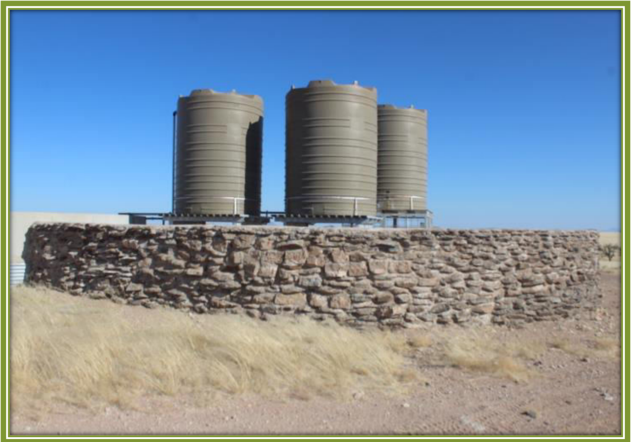
Figure 4: Existing boreholes with erected water storage tanks north of the mining claims; 73291, 73292,73293, 73294, 73295, 73296, 73297, 73298, 73299 and 73300, Khorixas District, Kunene Region.
