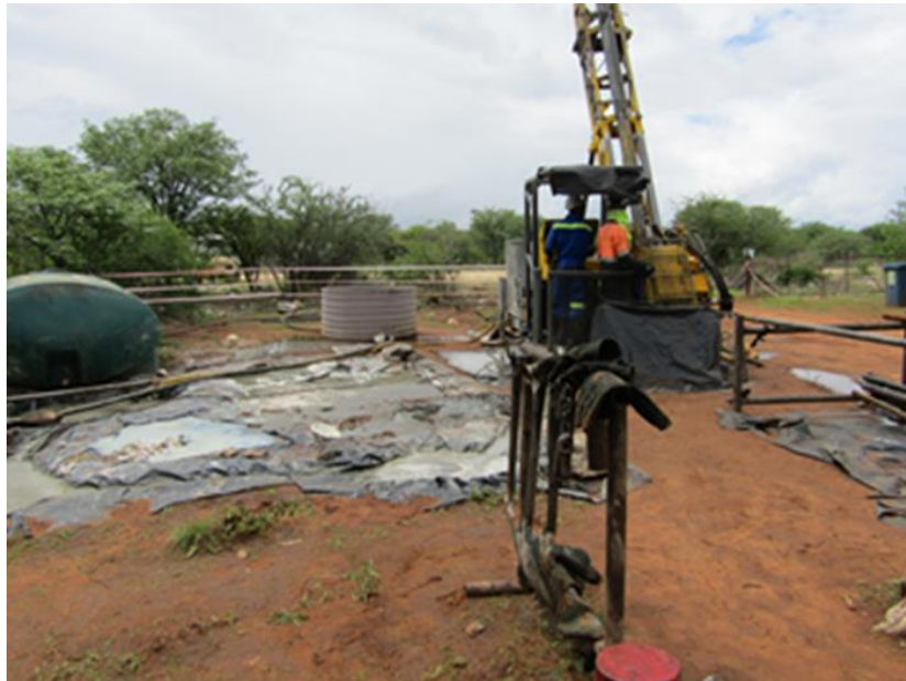
Figure 2 - Plastic lined sumps and drilling in progress
