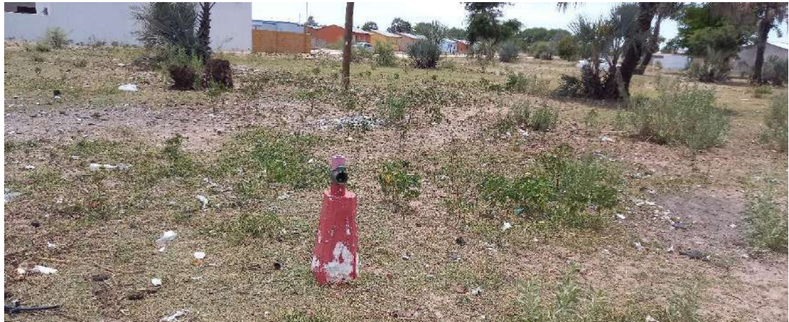
Figure 7: A Fire Hydrant Point
