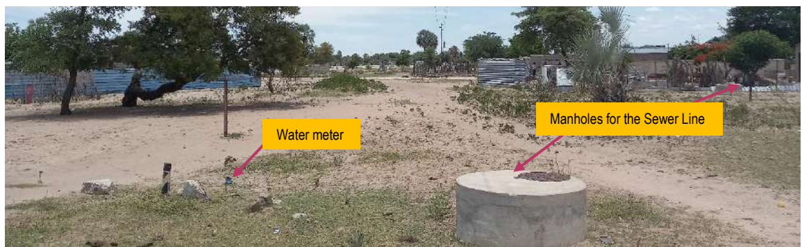
Figure 9: Manhole for Sewer Line Inspection
