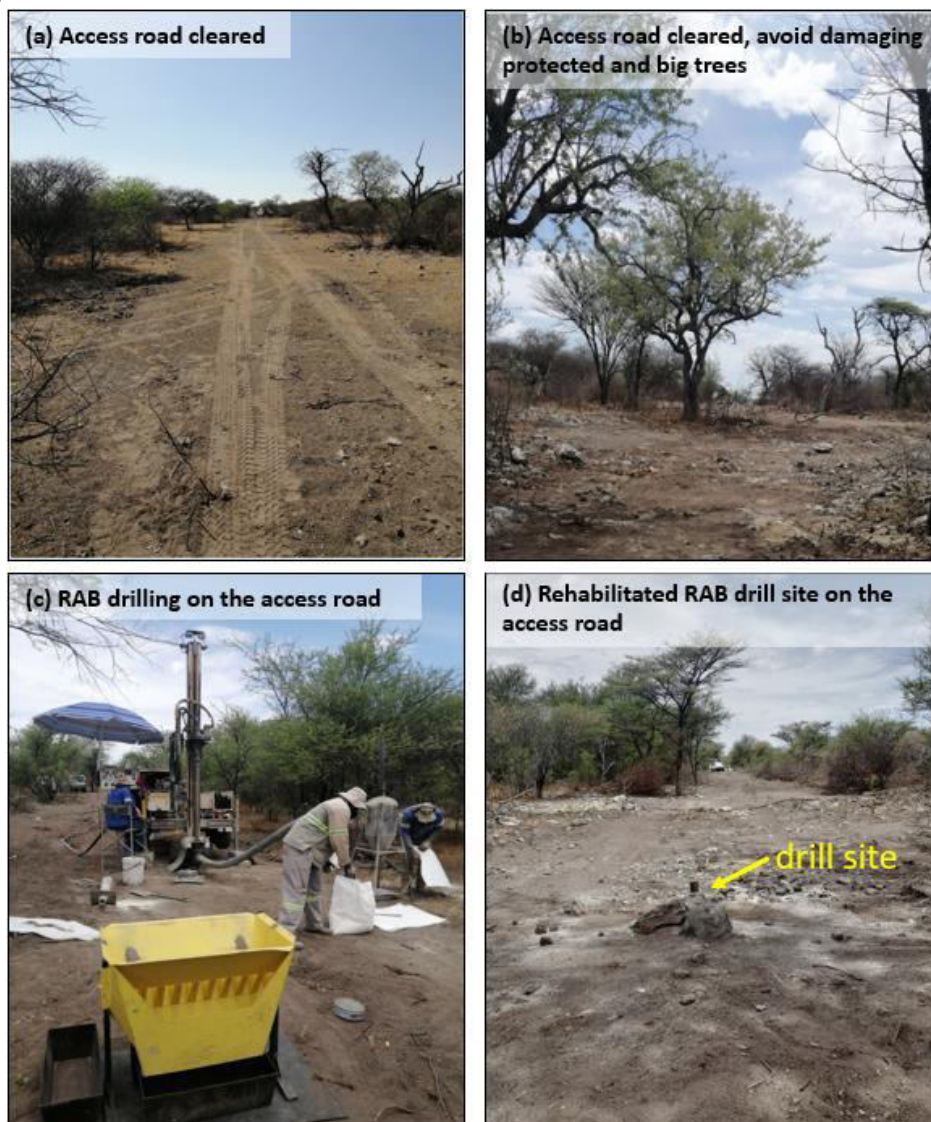
Figure 3 - Plates 1(a): Access road cleared, (b): Protected and big trees were avoided on the access road cleared, (c) RAB drilling on site and (d): drill site after rehabilitation from July to December 2020.
