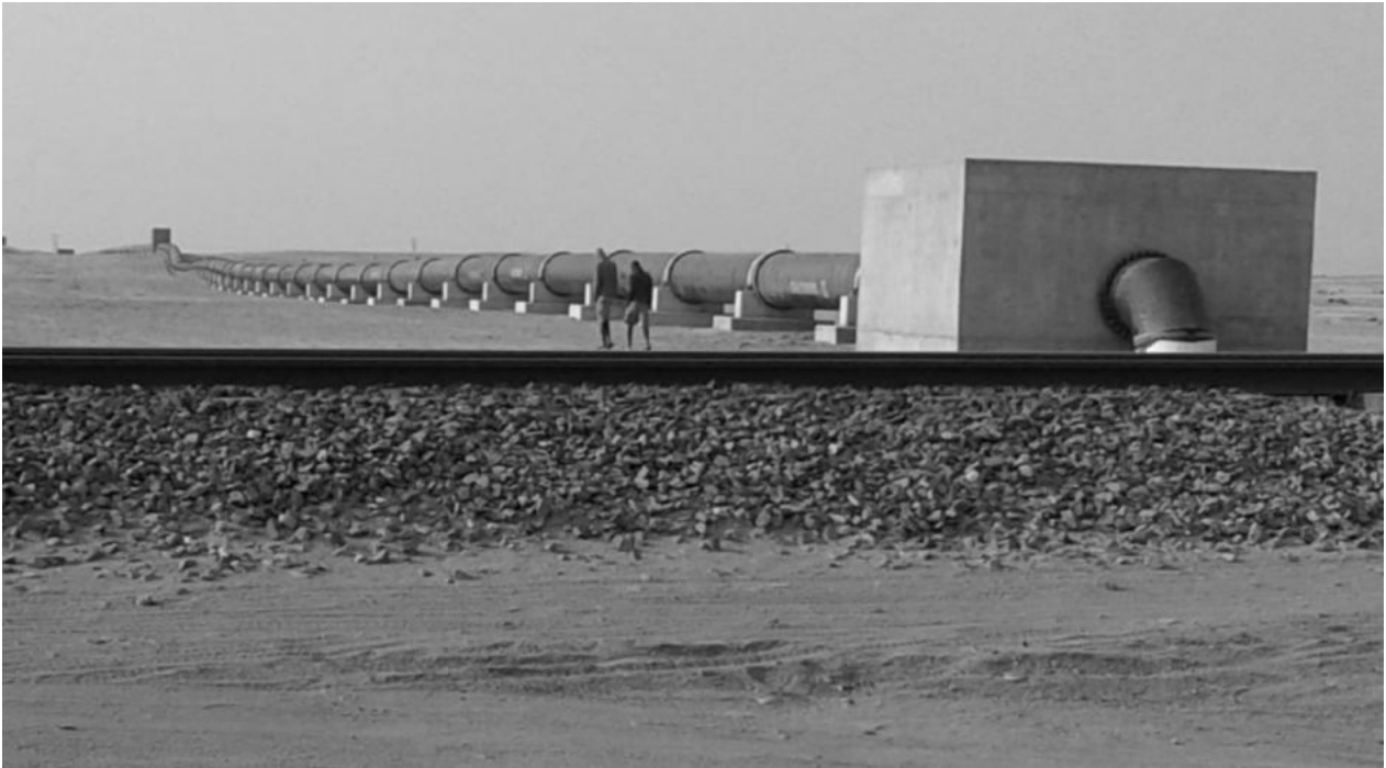
Figure 2 - Namwater pipeline from Areva Desalination Plant that crosses under the railway just east of Swakopmund (from: Hartz, C., 2017)
