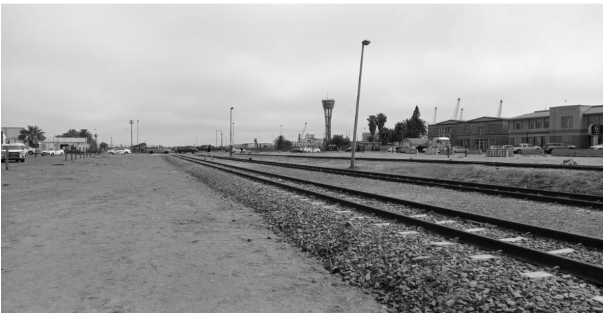
Figure 1 – Condition of the upgraded railway line (left) in comparison to the fuel line (far right), with NamPort in the background.
