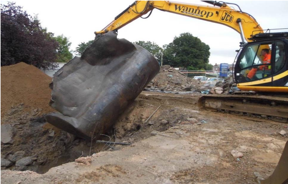
Figure 14: Former service station decommissioning
