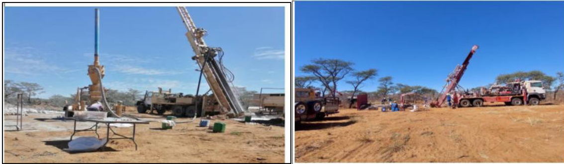
Figure 2-5: A drill rig on an EPL in the Omaheke Region (Resilient Environmental Solutions, 2022)
