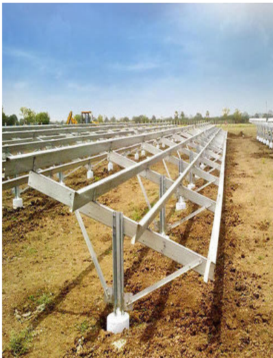
Figure 5: Completed PV Panel Mounting
