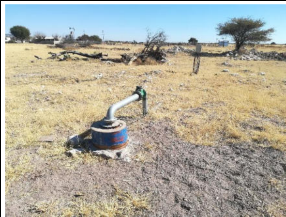
Photo 4-18 Typical borehole installation on Rika No. 266 (Portion 1)
