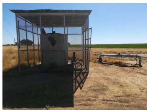
Photo 4-3. Fertilizer mixing tank
