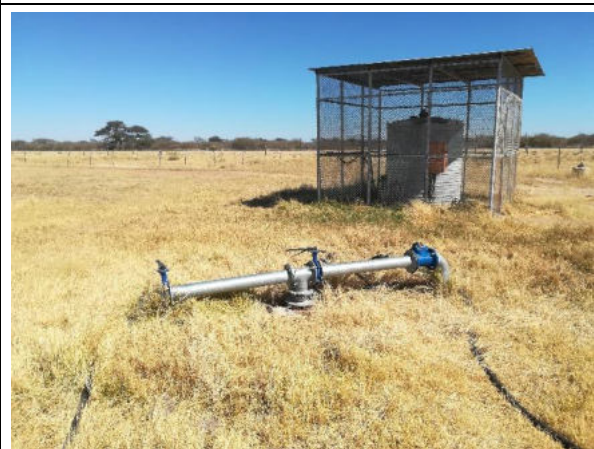
Photo 4-21. Borehole with flow meter and fertiliser mixer on the Farm Okatombaka
