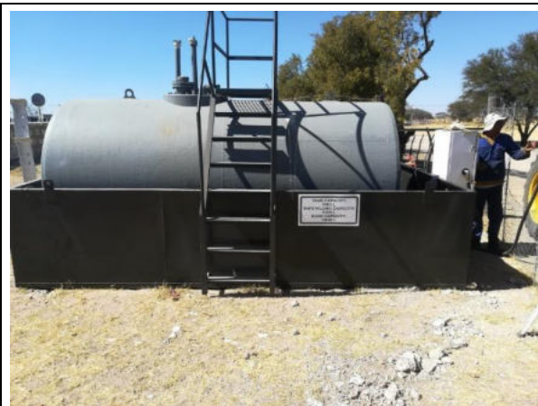
Photo 4-22. Diesel tank (9 m 3 )
