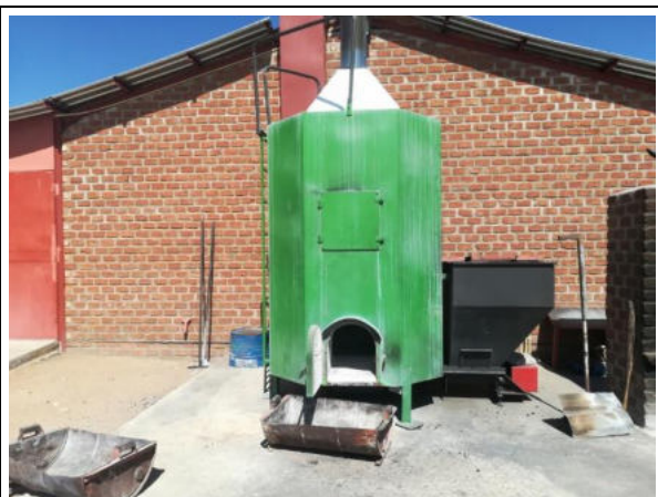
Photo 4-5. Drier room furnace
