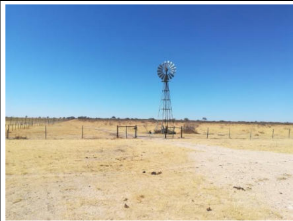
Photo 4-19. Typical stock watering borehole and installation on the Farm Okatombaka
