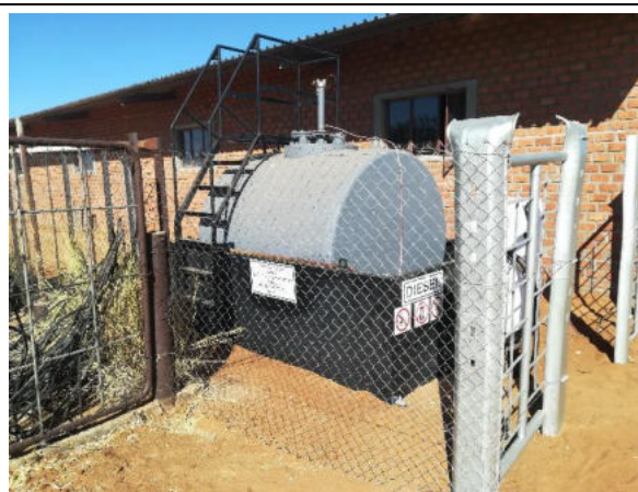
Photo 4-23. Diesel tank (4.9 m 3 )
