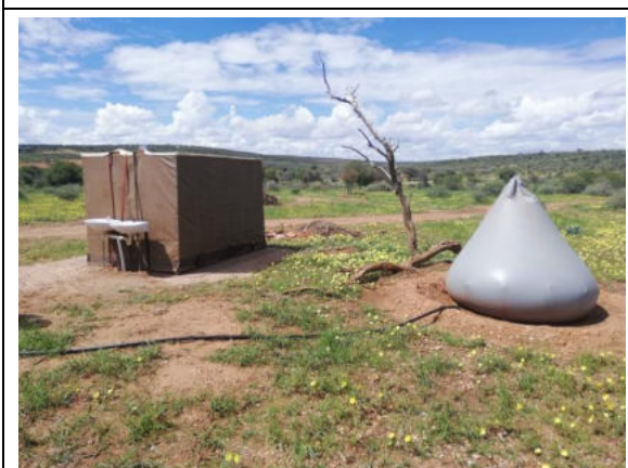
Photo 4-5. Water storage bladder
