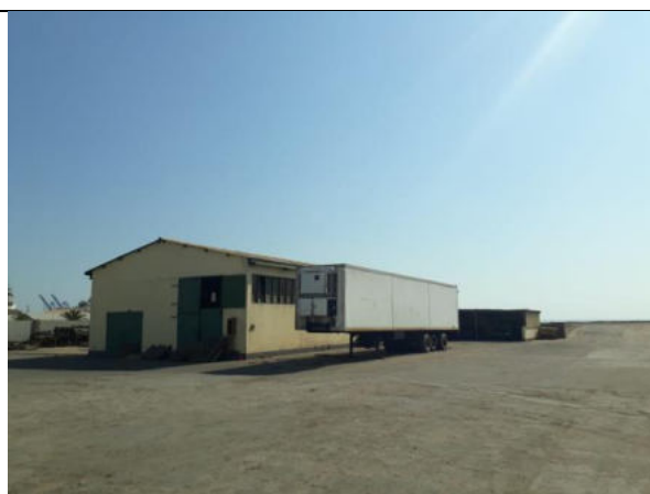
Photo 5-4 Old building to be demolished for new cold store construction
