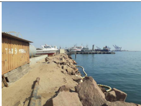
Photo 5-2 Area for new quay construction
