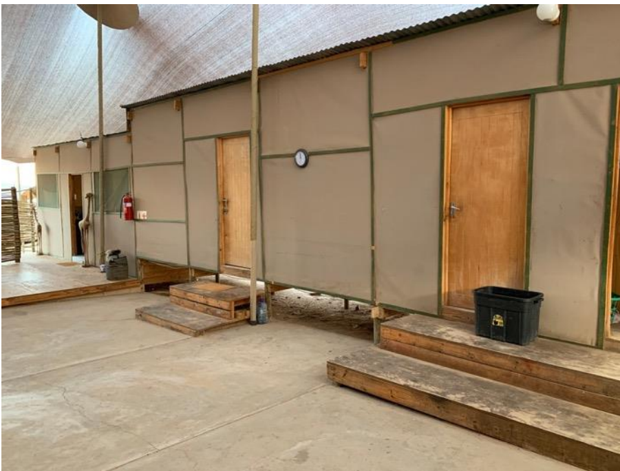
Figure 12. The office and store rooms inside the back of house building.
