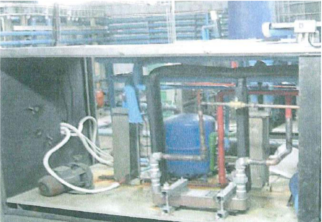
Plate 1.3: Example of the Heater and Chillers to ensure optimum water conditions at all times especially in the hatchery (Source: Atlantic Aquafarms (Pty) Ltd, 2015).
