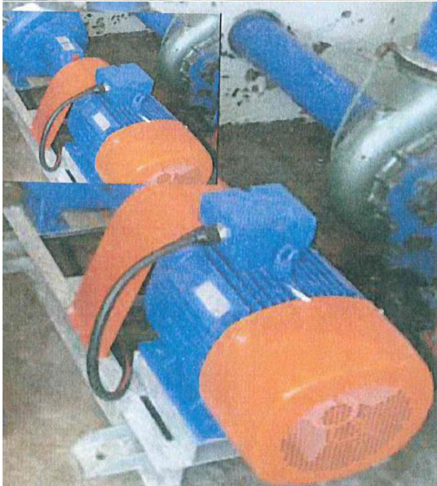
Plate 1.6: Examples of foam fractionators aerated by venture and also used for protein skimming (top photo) and main suction pumps (bottom photo) (Source: Atlantic Aquafarms (Pty) Ltd, 2015).
