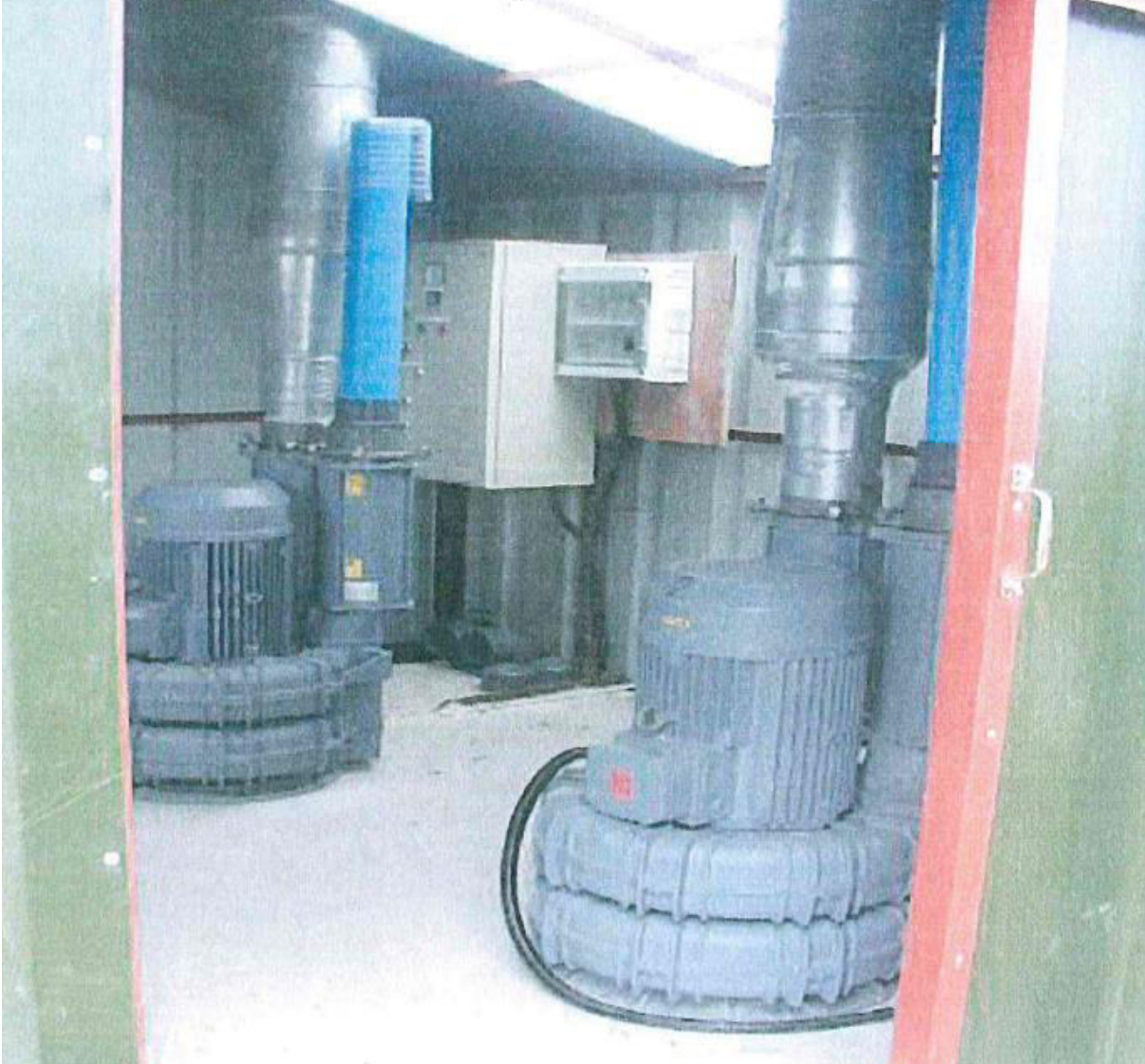
Plate 1.4: Example of the types of fans and blowers used to drive water and air circulation (Source: Atlantic Aquafarms (Pty) Ltd, 2015).
