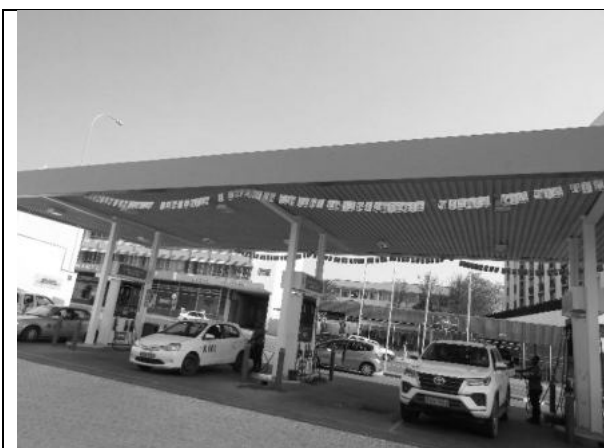
Image 1: A Canopy installed on site
