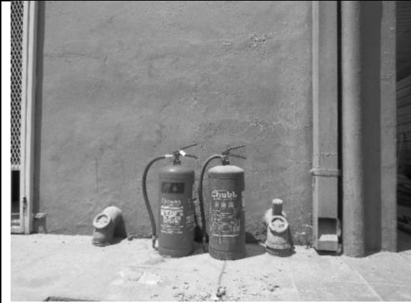
Image 1: fire extinguishers on site
