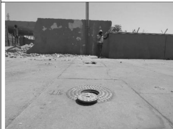
Image 3: concrete slab around the tanks filler area.
