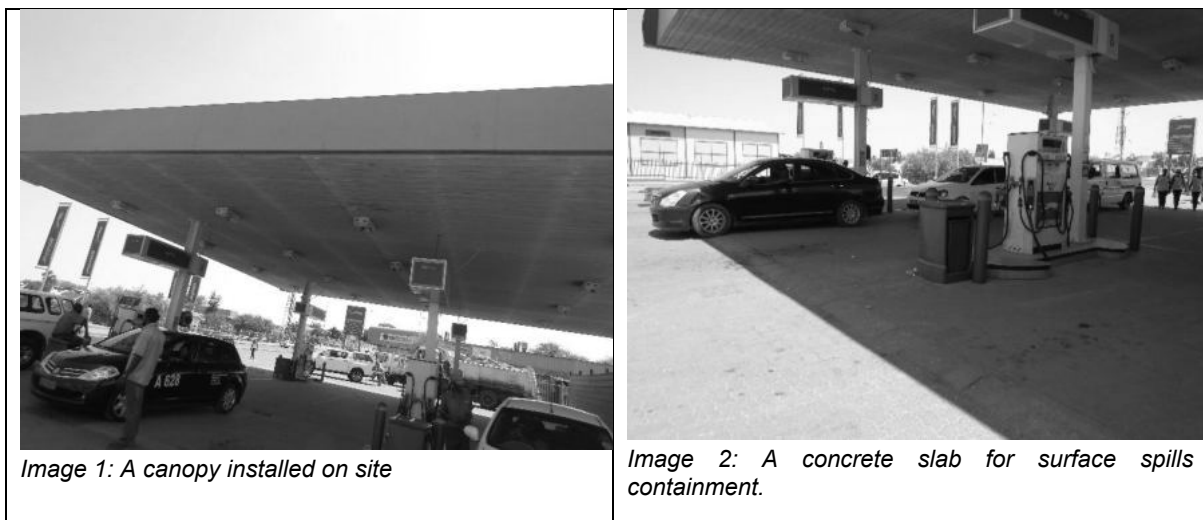
Figure 1: surface pollution control measures currently on site
