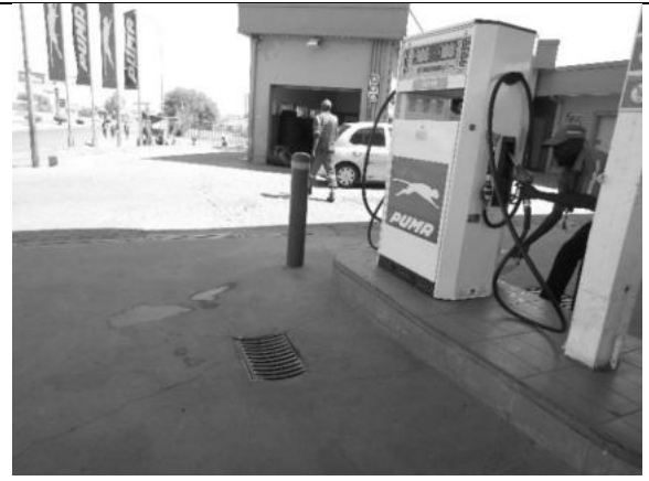
Image 2: A concrete slab at dispensing points and around tanks filler area for oil spill containment.
