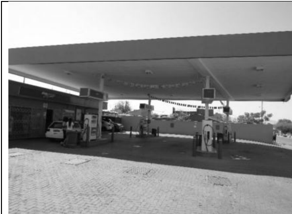
Image 1: A canopy installed on site.
