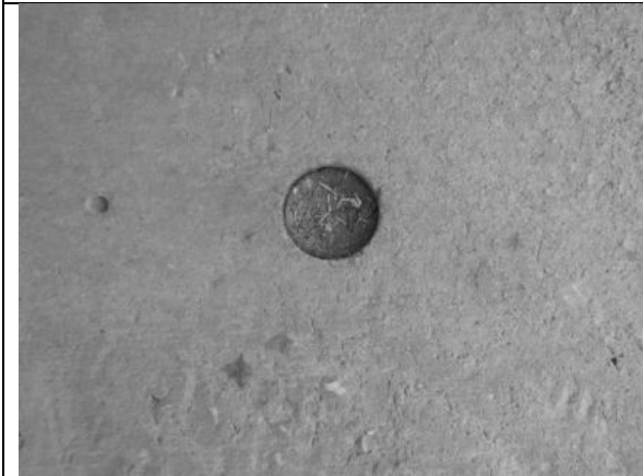
Image 3: Monitoring well on site.
