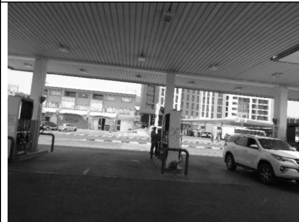
Image 3: Minor oil spills occurring on site, sand is used as an absorbent and remaining oils washed into the oil & water interceptor.
