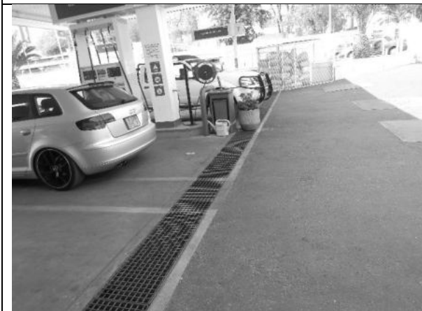
Image 3: Storm water drainage around the site, connected to municipal storm water reticulation
