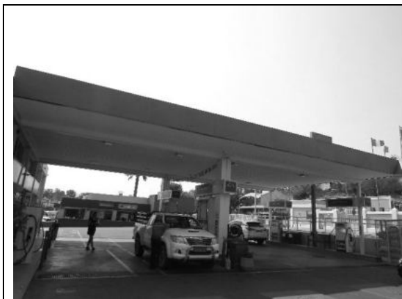
Image 1: A canopy installed on site
