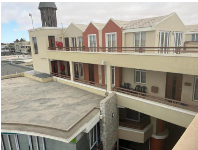
Figure 3: Tower - Opposite end of the Stadmitte building
