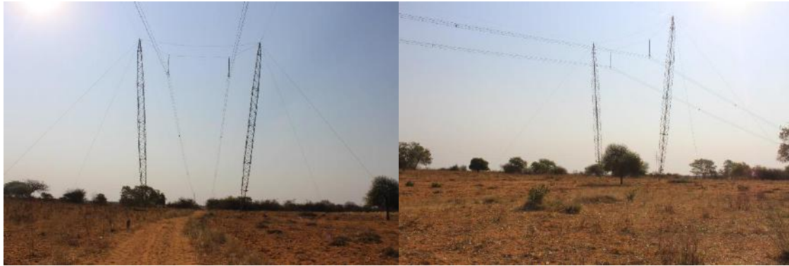
Figure 3: Powerline (Passing close to the project site)
