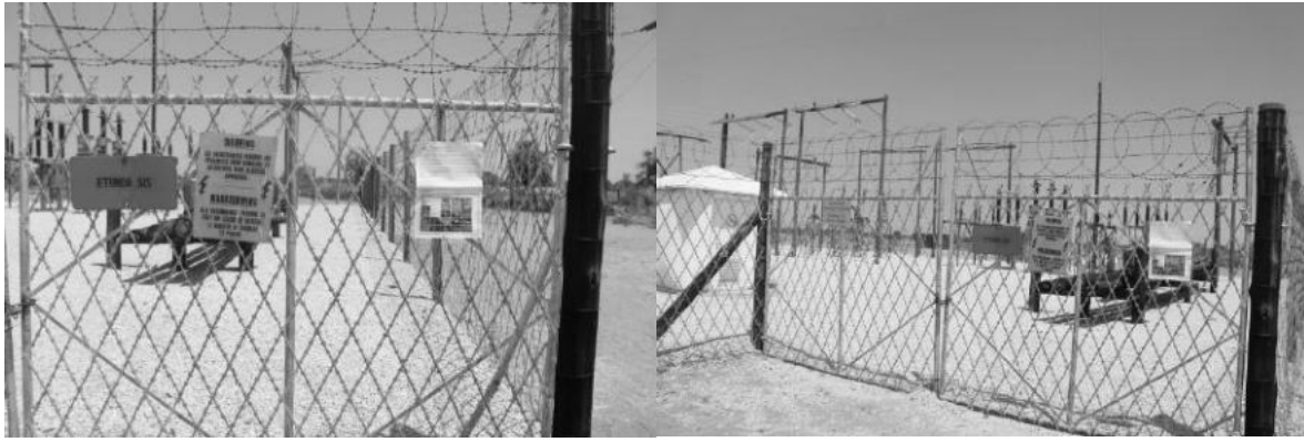
Figure 8: Site Notice- Etunda Transmission Station
