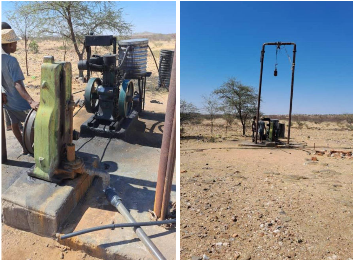
Figure 2-2: A photo of the existing borehole on Farm Sandamab Noord.
