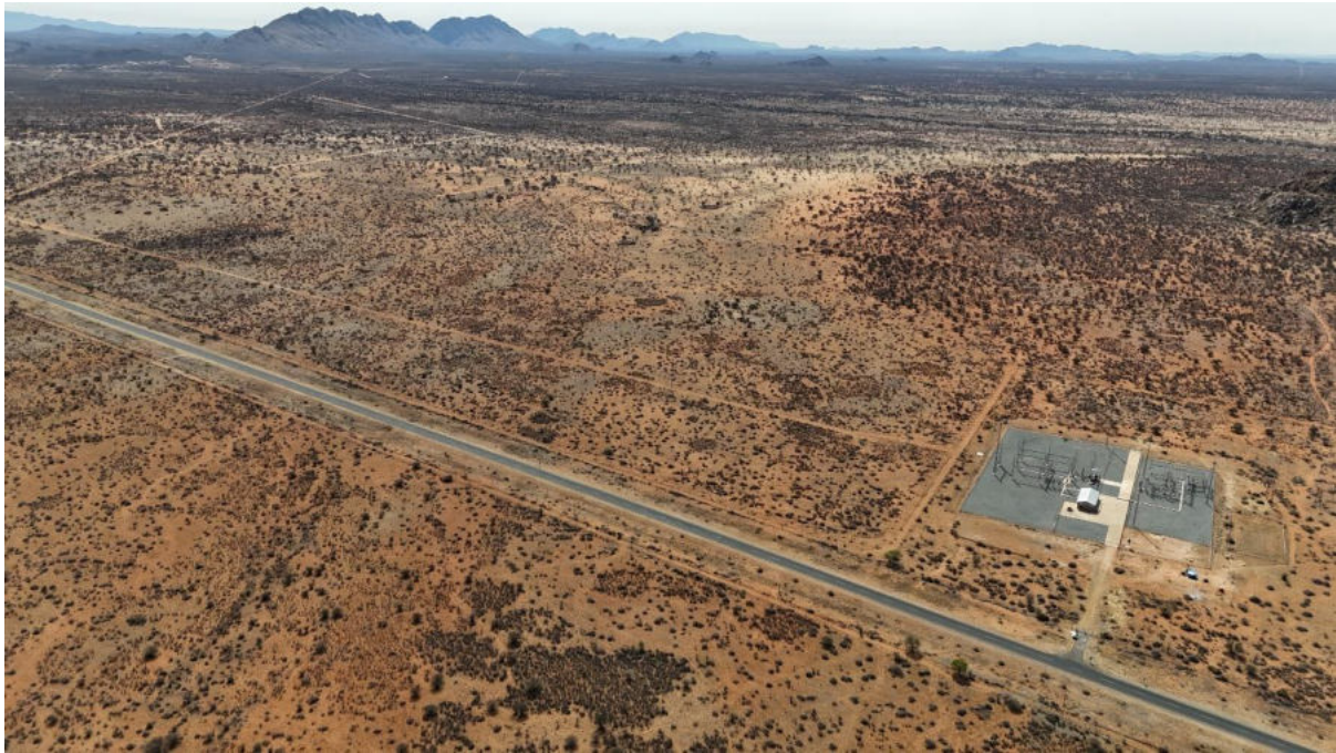
Figure 4. The Naruchas sub-station with the surrounding few outcrops.
