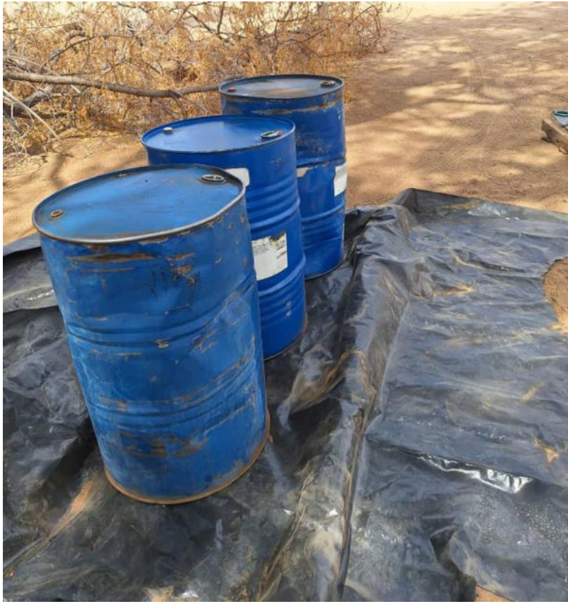
Figure 5 - Storage and utilization of hydrocarbons on plastic sheeting to prevent soil contamination.
