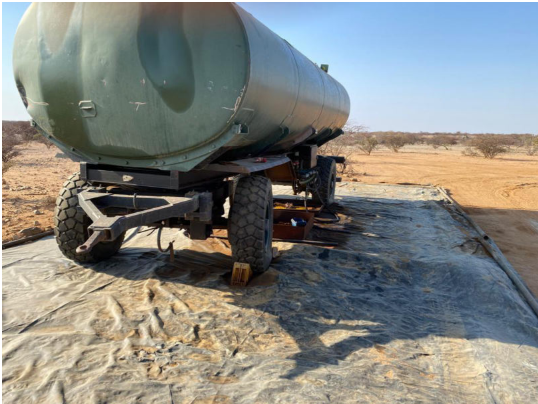
Figure 6 - PVC sheeting around diesel tank fuelling station in site
